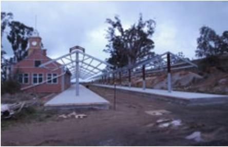
The exposed granite next to the platforms gives an idea of the challenges faced preparing the site for construction. Many truckloads of granite were removed after numerous explosions set by an explosives expert.
