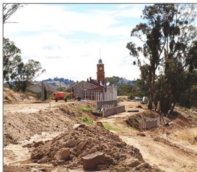
The three retaining walls will follow the curve of the tracks above, once they are in place. Roofing of the platforms has begun with the installation of batons under the stanchions.
