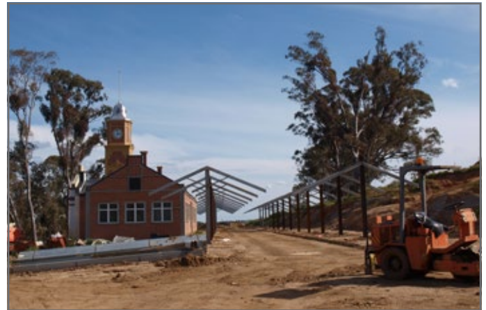
The new platform stanchions are ready for the platform roofing iron
