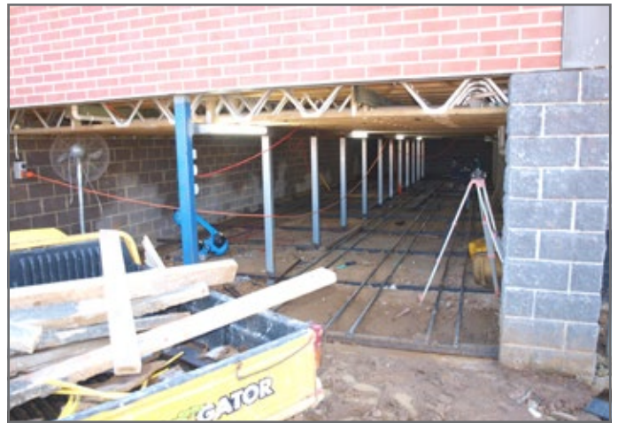
Space has been excavated below the Railway station for the storage of engines and the laying of six sets of tracks has commenced.
