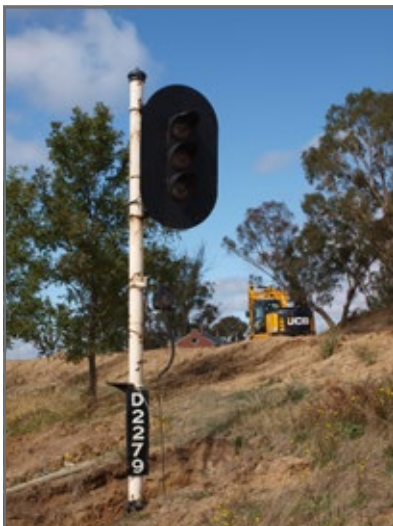
The first set of signals has been installed.
